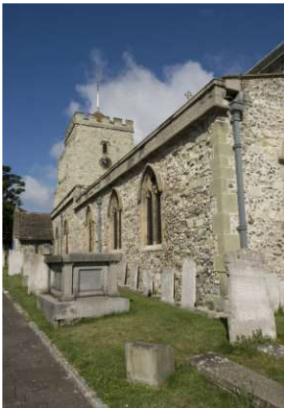
Fig. 3. St Mary's church: view from the south-east.
