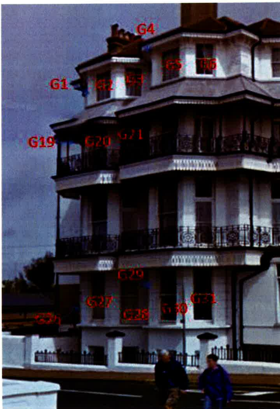
Photograph 5: Prior to works photos of East Elevation facing St Aubyn's Road (1)
