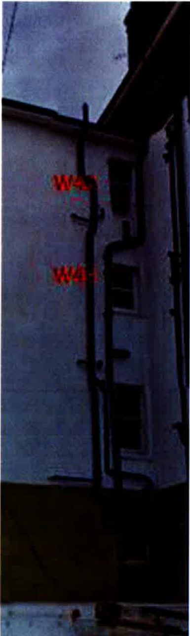
Photograph 2: Existing east elevation of building facing St Aubyn's Road (2)
