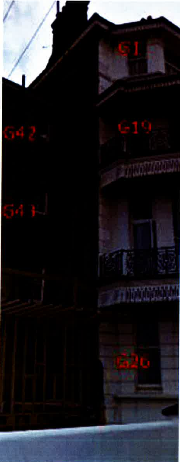
Photograph 6: Prior to works photos of East Elevation facing St Aubyn's Road (2)
