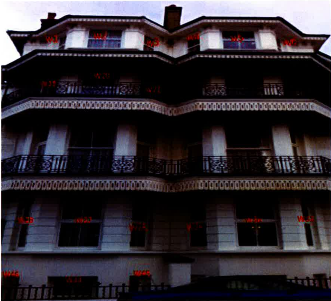
Photograph 1: Existing east elevation of building facing St Aubyn's Road (1)
