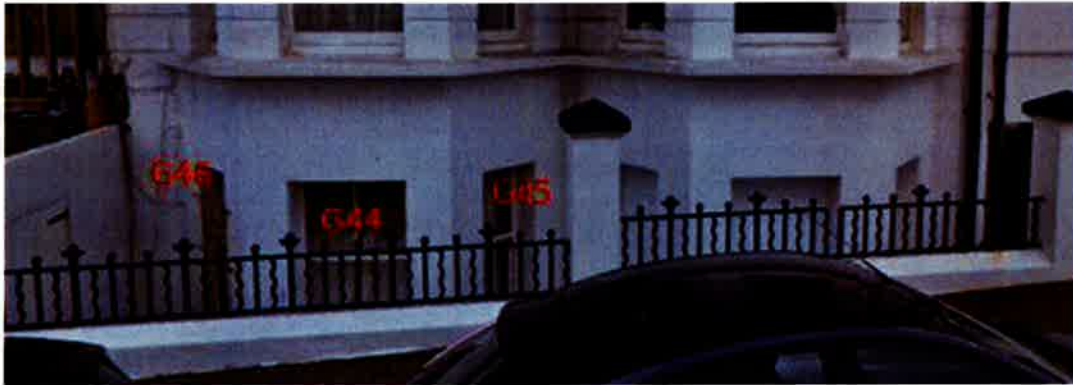
Photograph 8: Prior to works photos of East Elevation facing St Aubyn's Road (4)
