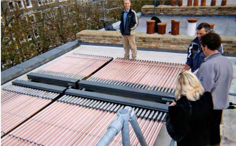
***A very large array of evacuated tube solar heaters installed on the flat roof of a large multi-occupied building in a conservation area (photo ECSC)***
