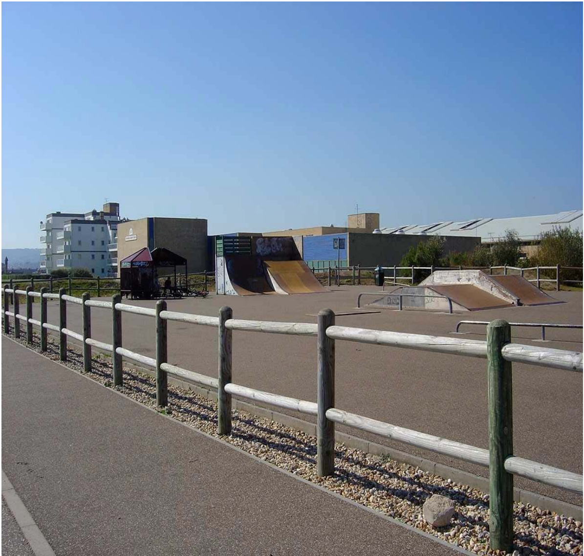
1. Oblique View to West Across Skate Park
