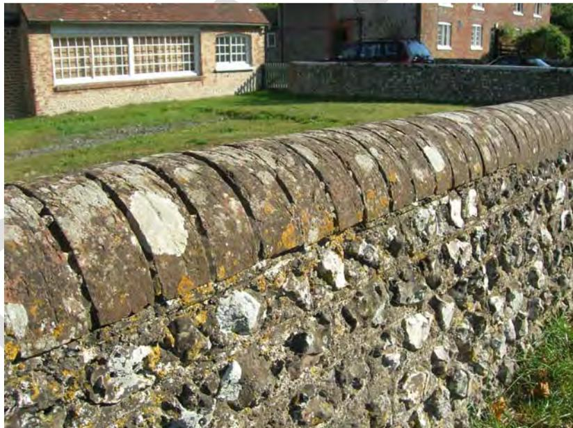
*Wall constructed of field flints with contrasting half round red brick coping*
