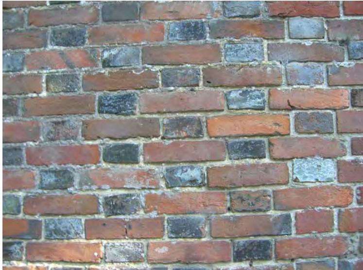
*Example of wall constructed of vitrified headers with red stretchers*
