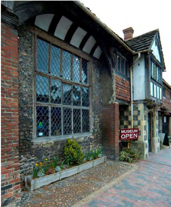
Fig. 29. Anne of Cleves House, Southover High Street.
