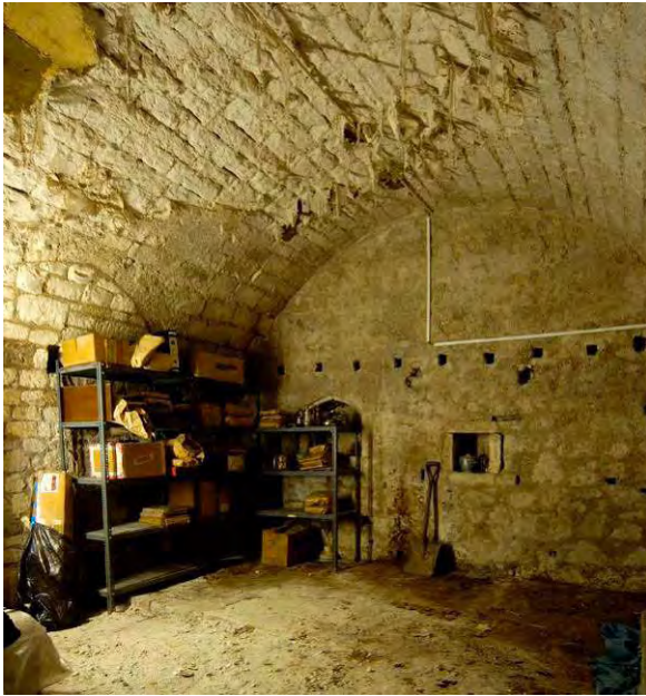
Fig. 27. 70-2 High Street: undercroft looking northwards, with blocked doorway on the left to adjacent undercroft (no. 73).
