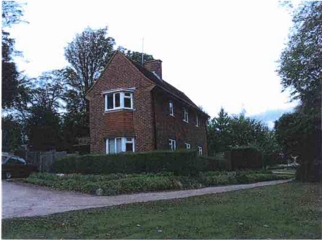
1. Manor Gardens Cottage from South East
