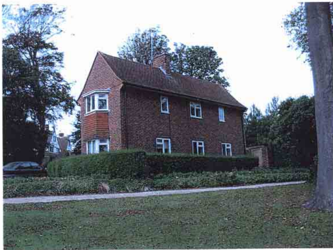
4. Manor Gardens Cottage from South East (2)
