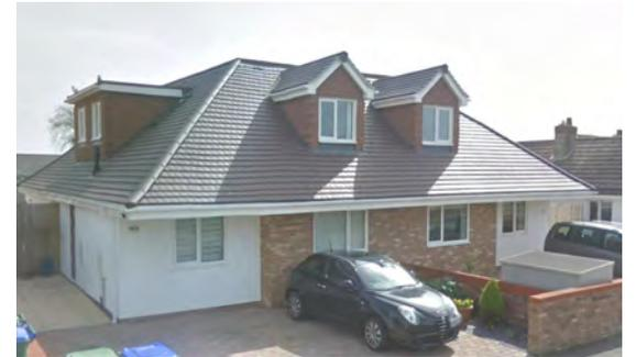
Figure 20. Example of bungalow with converted roof.
