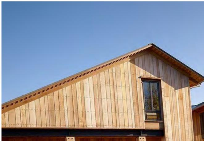
Figure 250. Example of a saltbox roof.
