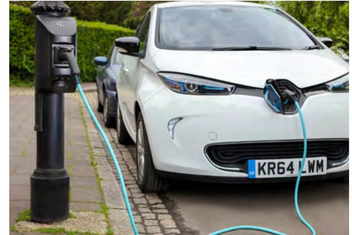
Figure 344. Public car charging point incorporated into the street design.
