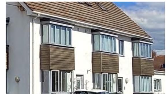
Figure 30. Example of poorly chosen materials that are easily weathered by the salt air.
