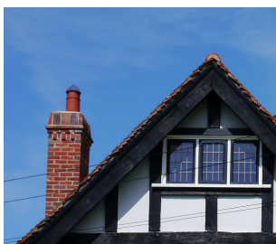
Gable ended roof
