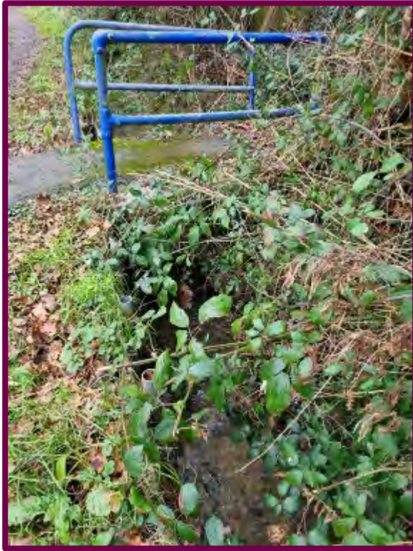
Figure 5. Culverted channel beneath footbridge (inlet)
