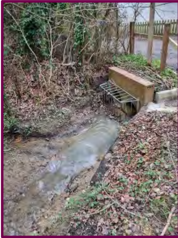
Figure 3. Culvert inlet beneath Eastern Road, two culverts with trash screen
