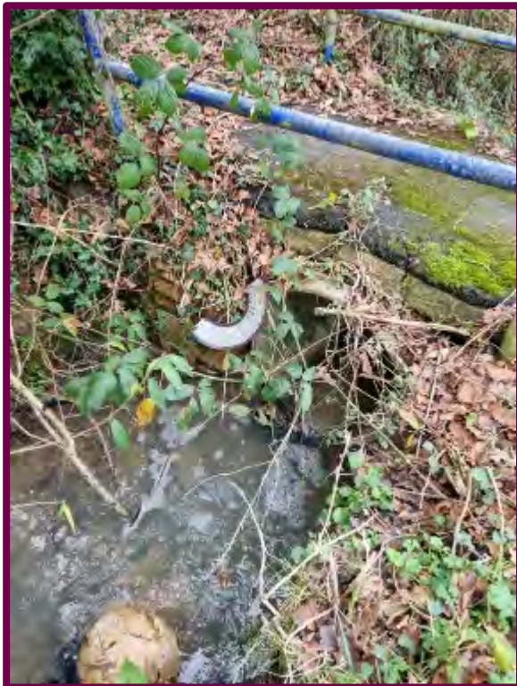
Figure 6. Culverted channel beneath footbridge (outlet)
