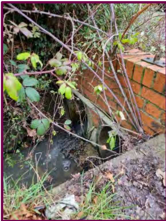
Figure 4. Culvert outlet – two culvert outlets
