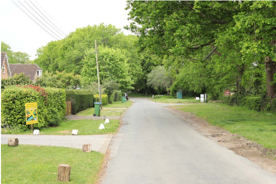
F. Further from the Green Road junction, Eastern Road retains the character of residential frontage and amenity space.
