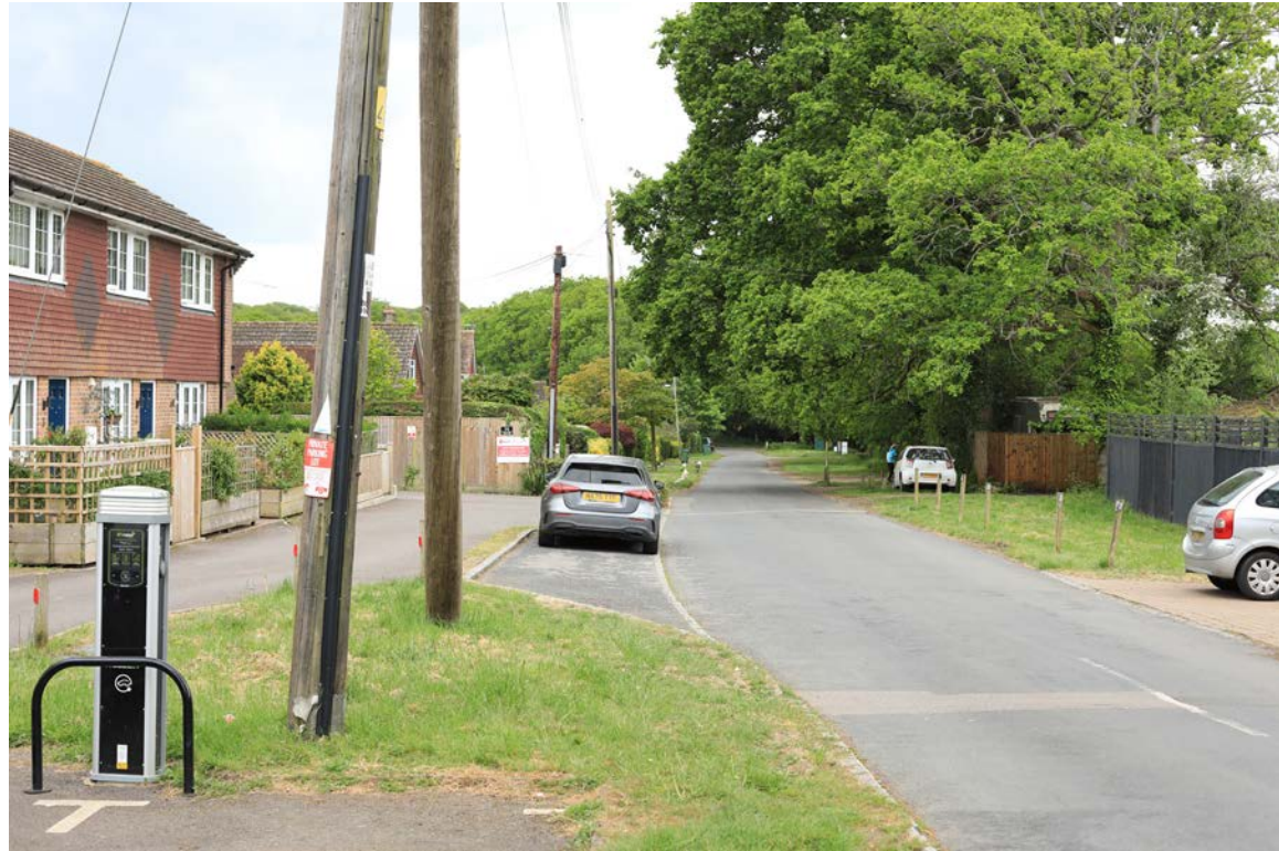
E. View from Eastern Road along the route of the Sussex Border Path through the settlement.
